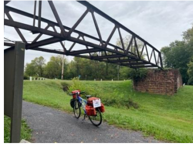
This abandoned bridge crosses the Canal at White's Ferry
