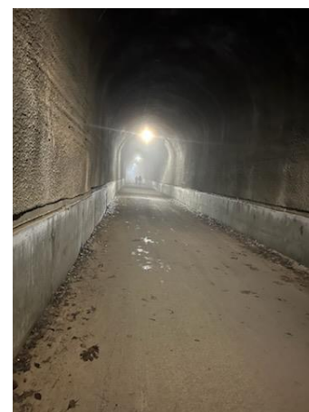
Inside Mount Savage tunnel looking toward where I was
