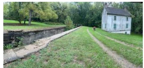
A typical Canal lockhouse and canal trail
