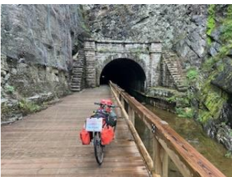
East entrance to the Paw Paw tunnel
