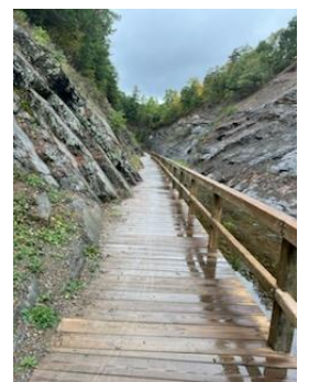
Another view of the tunnel approach from the east.
